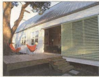
OUTSIDE-IN: A deck off the home's central breezeway "extends" the living room when the weather is nice.
